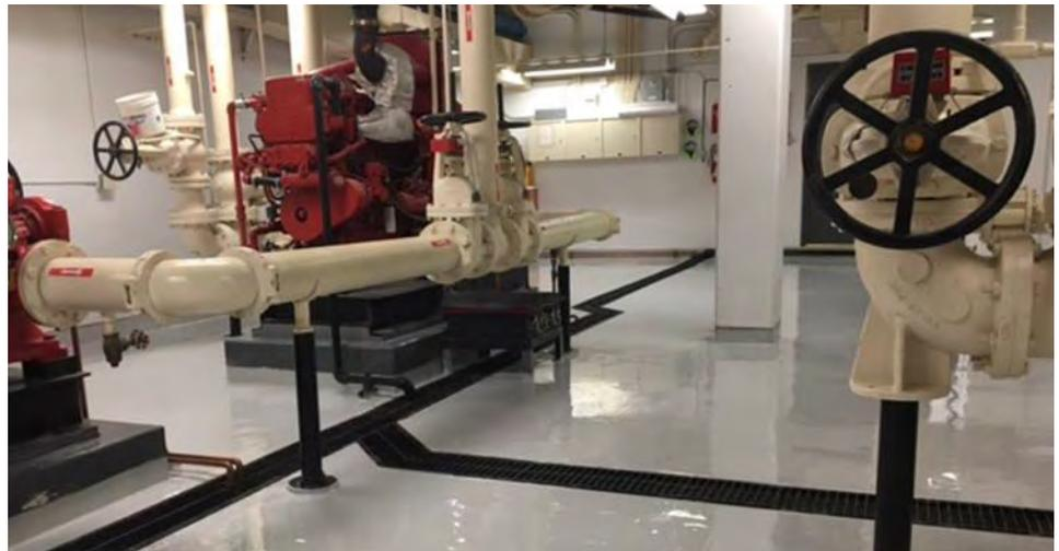
In January, we completed the 5-Year Standpipe/Sprinkler system inspection and testing. This inspection and testing is required by the National Fire Protection Association (NFPA) and the California Code of Regulations (CCR) Title 19; Public Safety.
